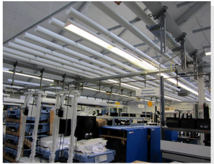
Montage horizontal T24-Schiene
